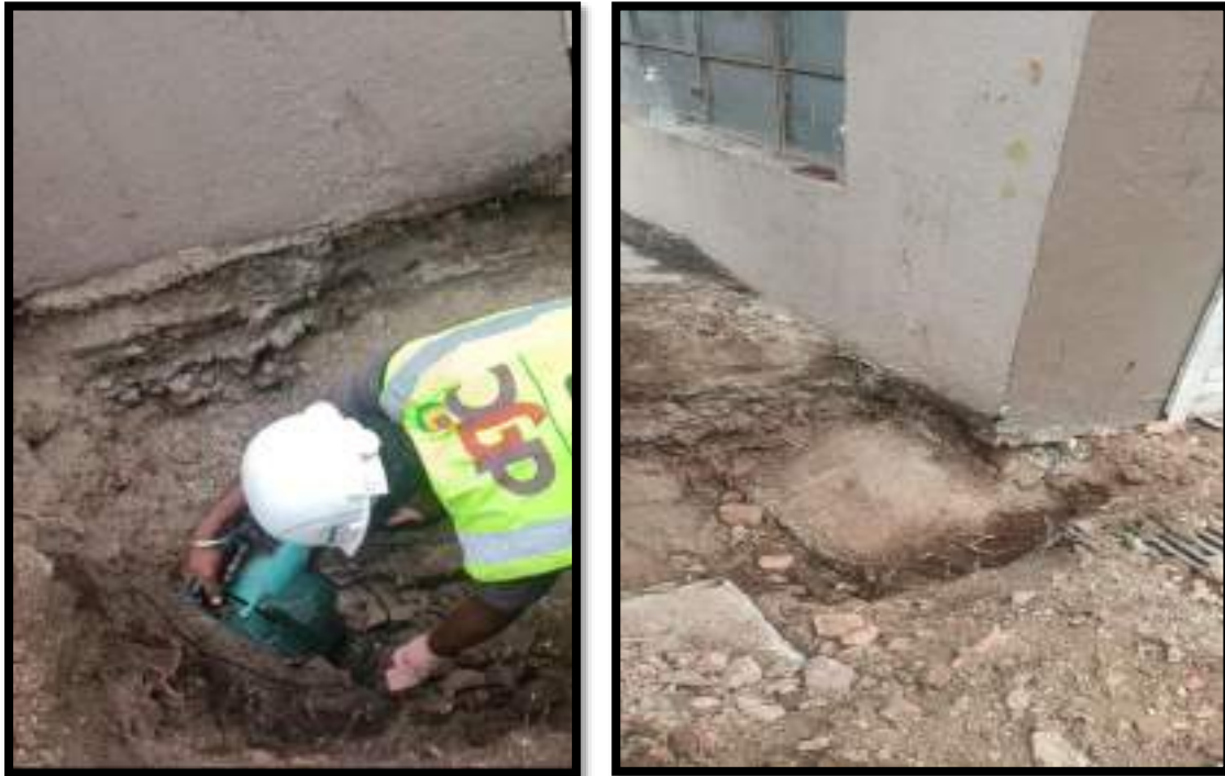
Figure 7.6: Exposing reinforcement for foundation analysis
